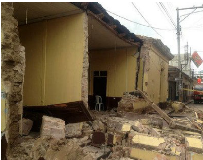
Terremoto en San Marcos, Guatemala http://www.telesurtv.net/articulos/2012/11/07/aumentan-a-39-los-muertos-por-terremoto-en-guatemala-9573.html
