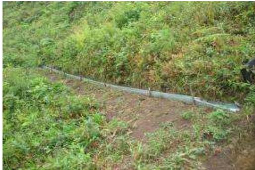
**Figura 9 Canal colector**
