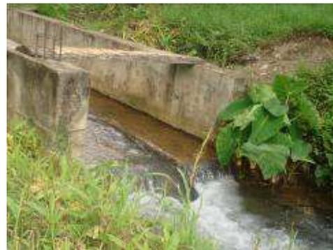
**Figura 30 Canal colector**
