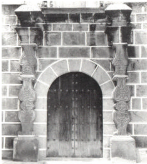
Fig. 104. Escuela de Cristo, Convent, Entrance, Detail, door and pilasters.
