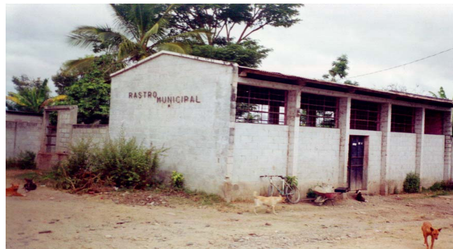
Foto No. 12 Fachada Principal
