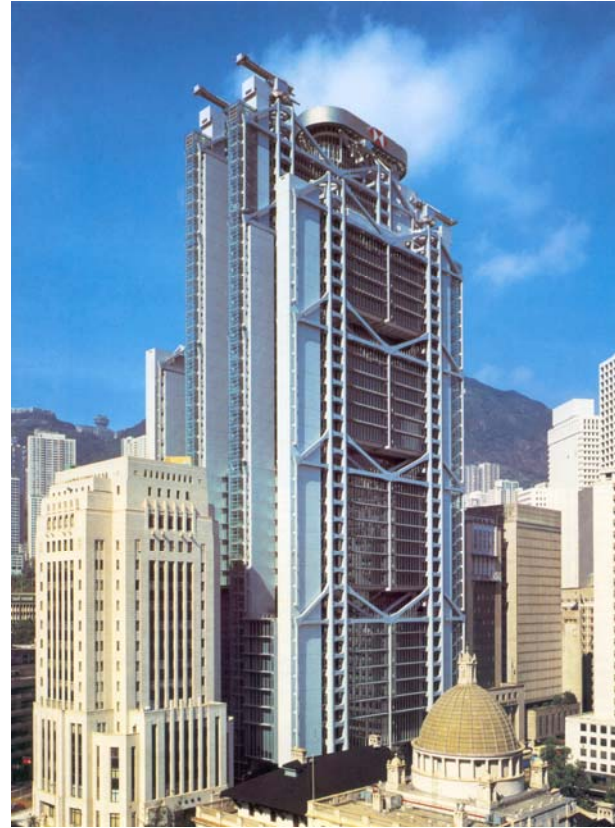
Ilustración II.33. Edificio central del Hongkong and Shanghai Banking Corporation, Hongkong, 1979-1986. Foster Associates (arq.), Ove Arup and Partners (ing.)
