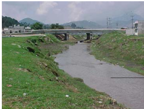
IMGAEN 18: PUENTE VEHICULAR
