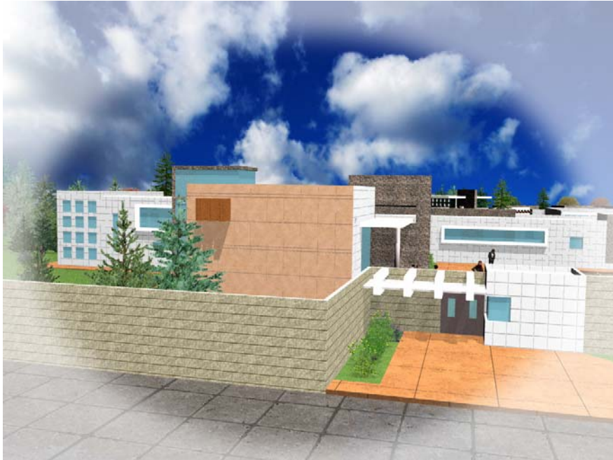
1 GARITA DE CONTROL PEATONAL
