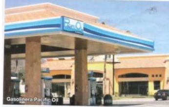
Gasolinera Pacific Oil
