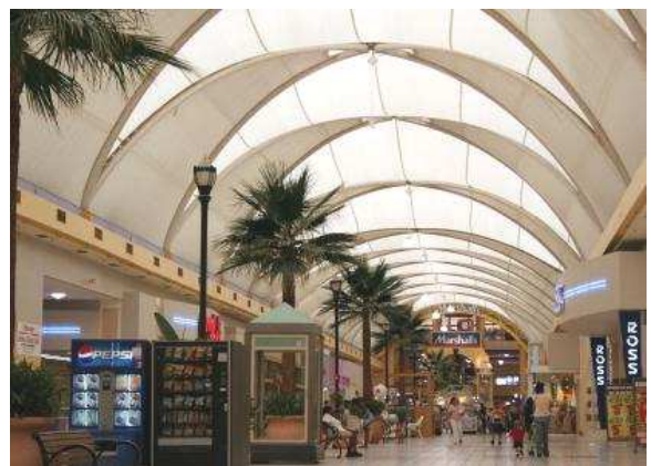
Imagen 103 Mall at 163rd Street, Miami
