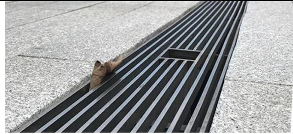
Figura No. 53 rejilla de drenaje para estares interiores de perros Fuente: <https://spanish.alibaba.com/product-detail/stainless-steel-linear-drain-kitchen-bathroom-shower-room-floor-drain-wedge-wire-grate-60498123474.html>
