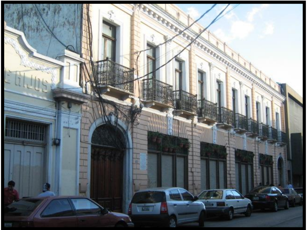
Fachada “Casa Larrazábal”
