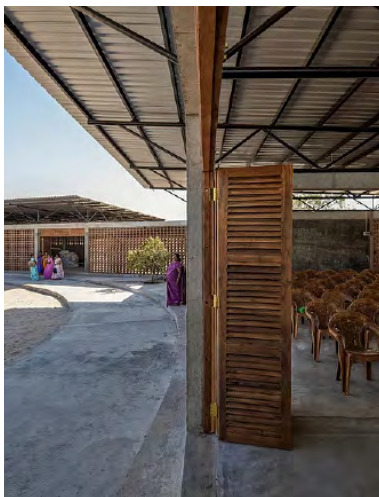
FIGURA 23 Sistema constructivo de los módulos, Fuente: https://wienerberger-building-solutions.com/expertise/lanka-learning-centre-sri-lanka-
