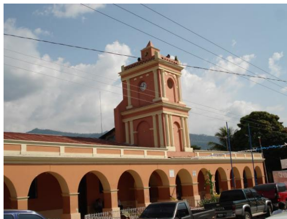
Figura 16: Vista exterior municipalidad de Quezaltepeque. https://mapio.net/pic/p-39118990/
