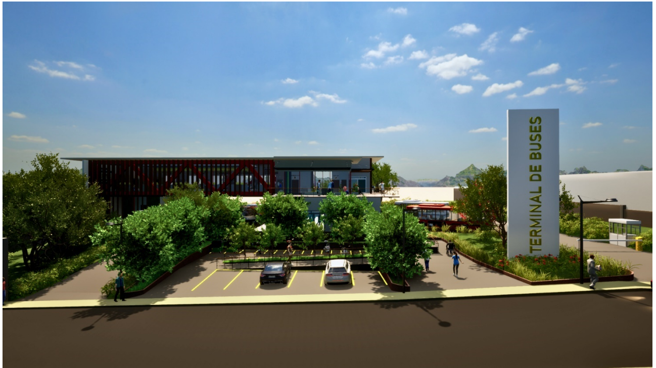
TERMINAL DE BUSES VISTA FRONTAL
