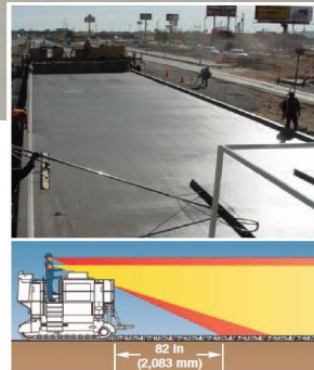
Increased visibility of slab behind paver.
