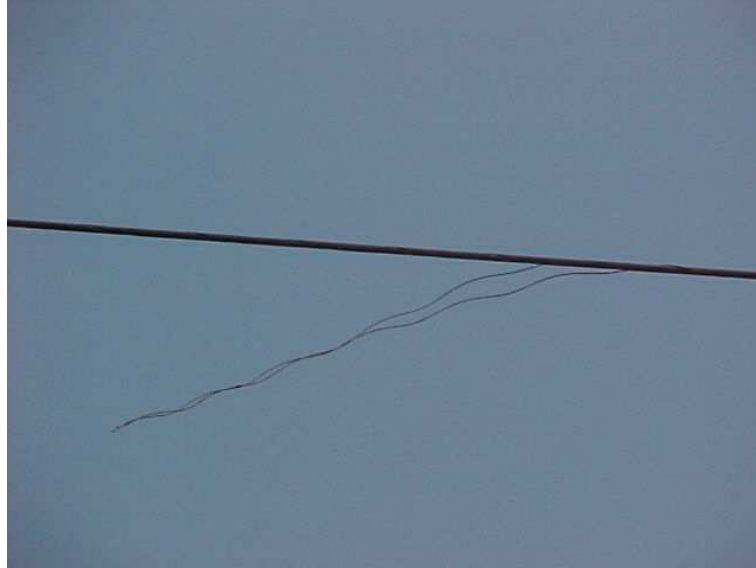
Figura 18. Conductor deshilado
