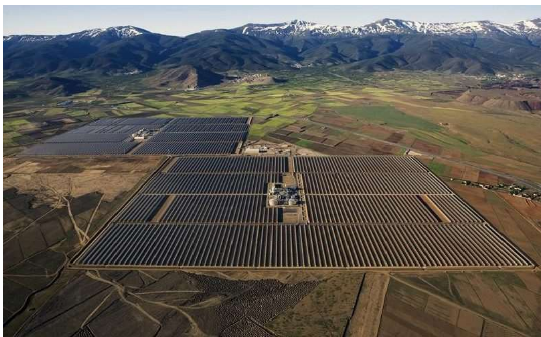
Figura 25. Central termosolar CCP
