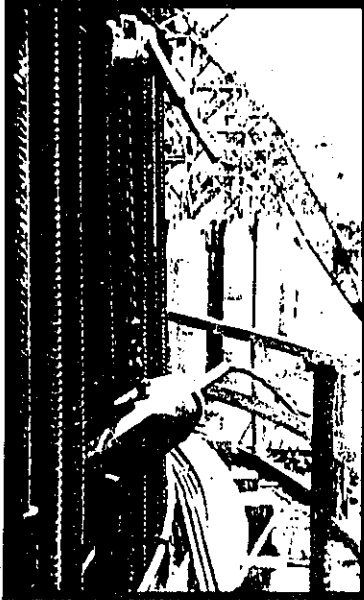
Bar-Grip BG1157 press supported from horizontal bar using comealong.
