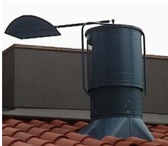
Figura 9. Extractor Venturi
