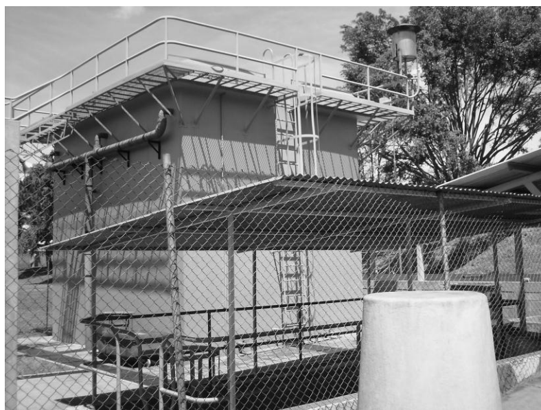
Figura 7. Reactor UASB
