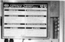
The "SERVICE-SAVER" enclosed electrical control unit is sealed from debris such as dust and moisture and is accessible through a side swinging door making the unit easily field serviceable.
