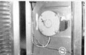
A side swinging door design gives EASY ACCESS to internal components like the "Super-Saver" control unit and blower motor, making it one of the easiest to service heaters on the market.
